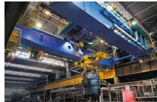
Ladle transport cranes 390/60t x 40m ©Photo: thyssenkrupp Steel Europe AG
