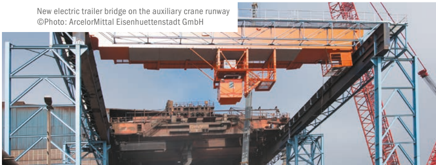
Erected auxiliary crane runway in a demountable design ©Photo: ArcelorMittal Eisenhuettenstadt GmbH
